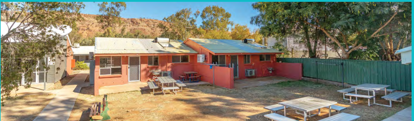
Transitional housing units at 34 South Terrace, Alice Springs
