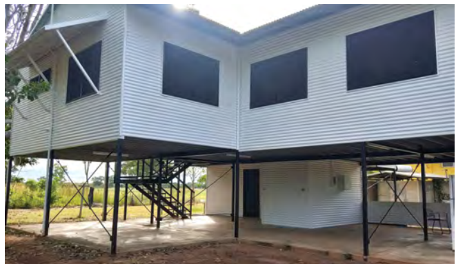
Completed works by Kalano Community Association in Miali Brumby community
