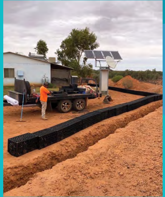
The new septic system being installed at Alice Well
