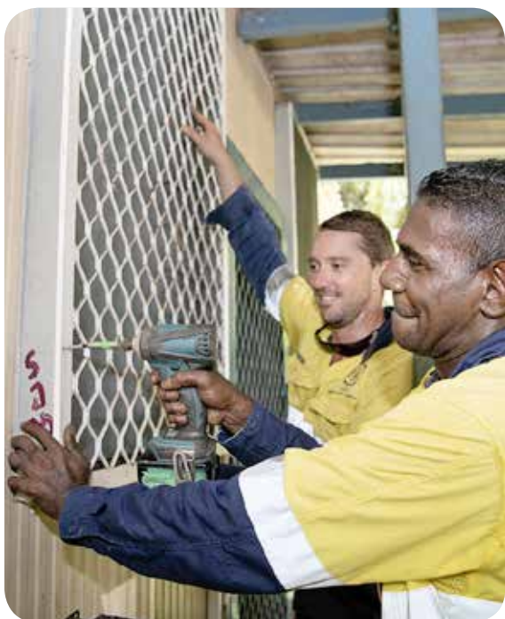
Contractor work in Angurugu
