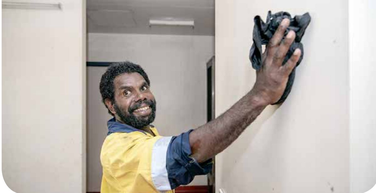
Contractor working on a home at Wallace Rockhole
