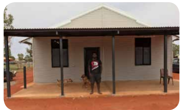
Newly constructed three-bedroom house at Ampilatwatja
