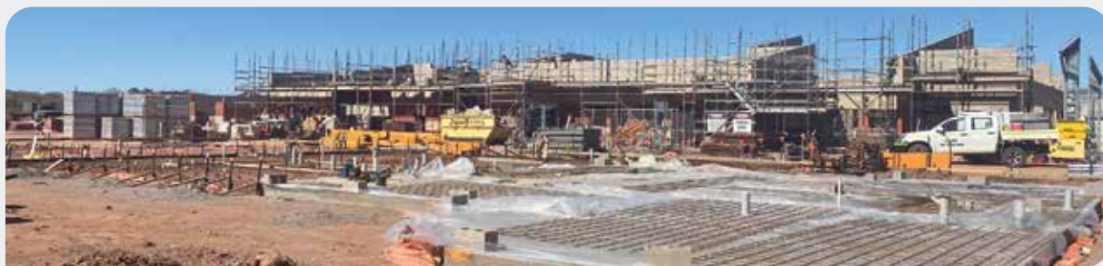
Construction at Alice Springs Youth Justice Centre.
